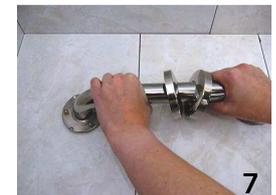
7. Remove the grab bar from the adapters again by removing the screws and spacers. If you are mounting horizontally or vertically, remove the screws and spacers on the lower end first to prevent potential injury. After removal of all screws and spacers, the adapters are now fixed to the wall in the proper location (see pic. 8).
