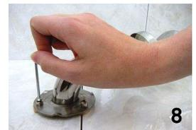
8. To open the black adhesive tube, carefully pierce the seal with the pointed end of the red tube key (see pic. 9).
