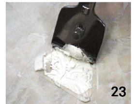
**Caution!** Use care not to scar the surface with the grips or razor knife when removing the adapter.
